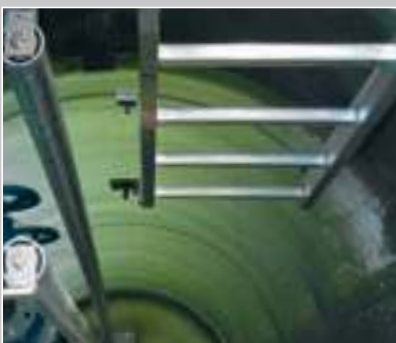
Built-in service ladder.
