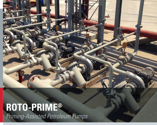
Roto-Prime® primingassisted centrifugal pumps are specifically designed for pumping petroleum products, petrochemicals and solvents. The Roto-Prime design incorporates a variable capacity vane pump which quickly and automatically evacuates air and vapor, making the pump ideal for loading and off-loading transports and stripping hoses.
