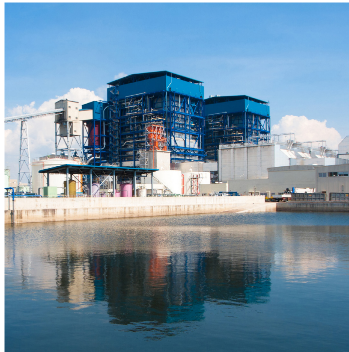
WASTE WATER TREATMENT
